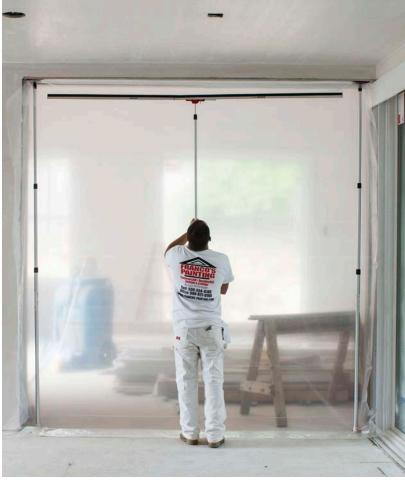
**TAPELESS SEAL RAILS & WALL MOUNTS**
