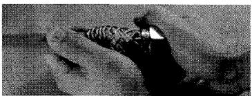
6. Slide nylon sleeve over conduit. Tapered end of sleeve should face compression nut (3/8" -1" sizes only).
