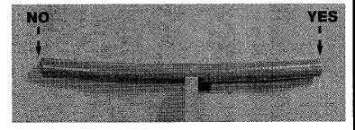
3. Compress the mouth or end of the grip expanding the mesh. Slip the grip over the end of the conduit.
