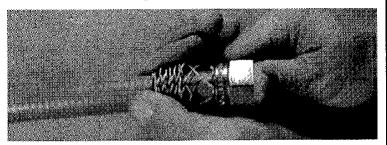
5. Compress the entire grip so that it expands and assumes a "Basket" appearance. With a rotating pushing motion, slide the conduit through the grip termination.
