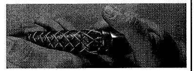
4. Slide the conduit through the grip to the first or second crossing of the wires.
