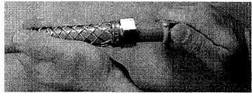
7. Insert octagon portion of ferrule into corresponding depression in the connector body. Slide the grip so it is tight against the ferrule and engage thread of connector. It is imperative that the compression nut be tightened to the positive stop provided by the shoulder on the body to provide a liquid tight seal. Smooth the mesh onto the conduit.
