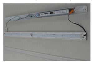
3. Ensure ground connection is made between channel and channel cover, and ensure that white wiring harness plug is snugly plugged in before channel is closed
